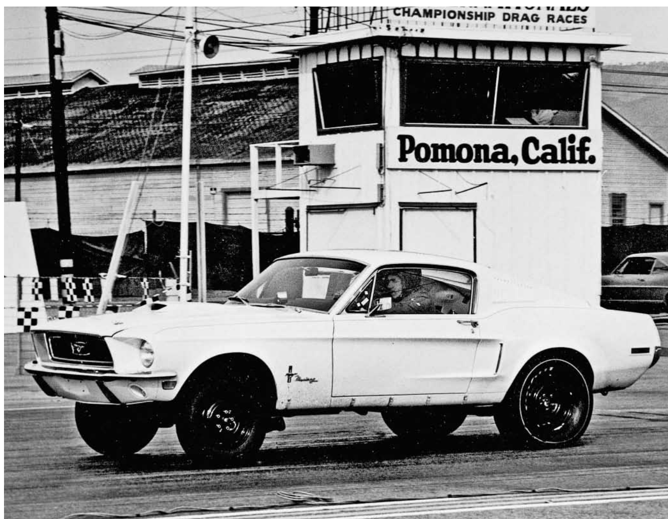
A special run of 50 Super Stock Cobra Jet Mustangs (all painted Wimbledon White) was built first, beginning in December 1967. These track-ready ponies weighed a little less than regular-production examples, as their insulation and sound-deadener materials were deleted.
