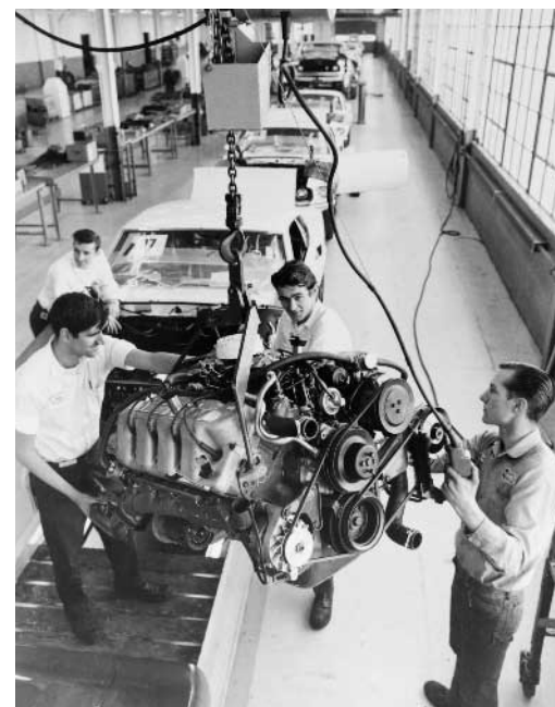
Above: The big Boss 429 V-8 was literally shoehorned between Mustang flanks at the Kar Kraft works in Brighton, Michigan.
